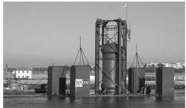
Fig. 2. Photo of the AWS pilot plant before submerging.
