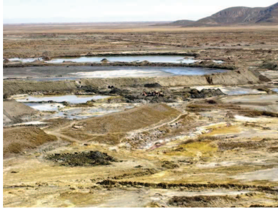
Leaking tailings dams at an artisanal mine, Lake Poopó Basin, Bolivia (Tobias Rötting)
