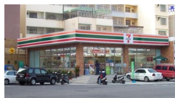
Figure 1: Convenience store façade.
